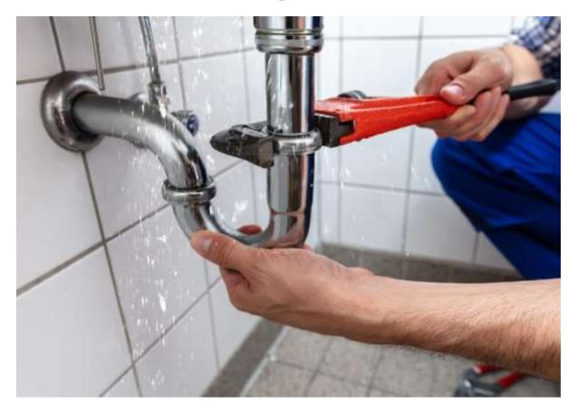
Installation of water pipes in a building is a complicated process and the material must be strong, durable, and resistant to corrosion <u>romanoplumbingutah.com</u> and should last longer. For ordinary water supply, we use material types like brass, copper, and stainless steel and for sewage supply, we use material types like steel, copper, cast iron, and asbestos cement.
